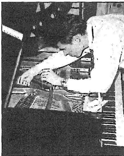
Photo 5 — Fitting hammers to strings with hook. Notice tray for voicing tools on stretcher.
